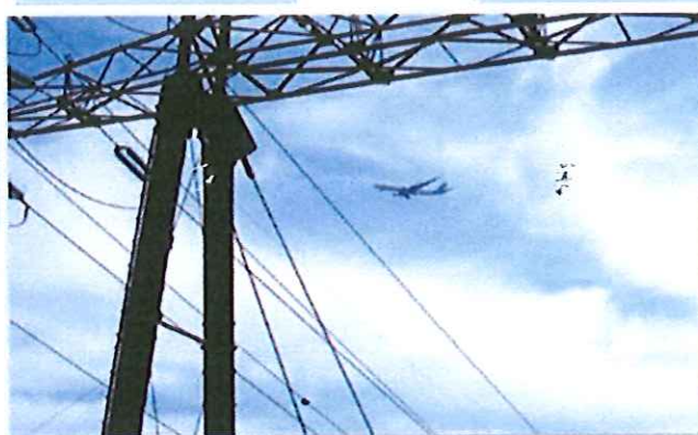
Filiform: Power lines, telecommunication lines, etc.
